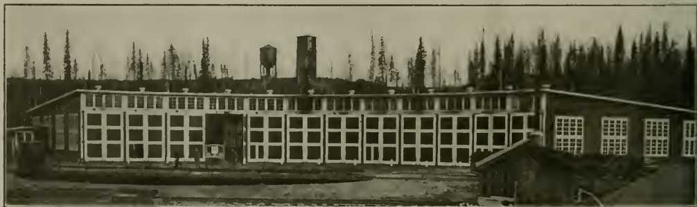
NEW SHOPS RECENTLY COMPLETED ON THE ALASKA RAILROAD.
